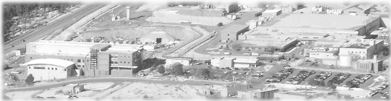
LANL’s Technical Area-55 with the plutonium pit production facility “PF-4” on the right and CMRR “Rad Lab” on the left, with the excavation for the future “Nuclear Facility” behind it. Photo: Scott Kovac, Nuclear Watch New Mexico
