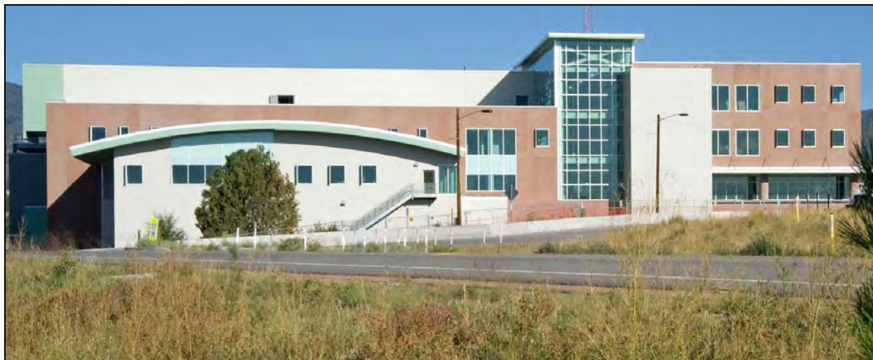
Figure 2-3 Radiological Laboratory/Utility/Office Building in Technical Area 55
