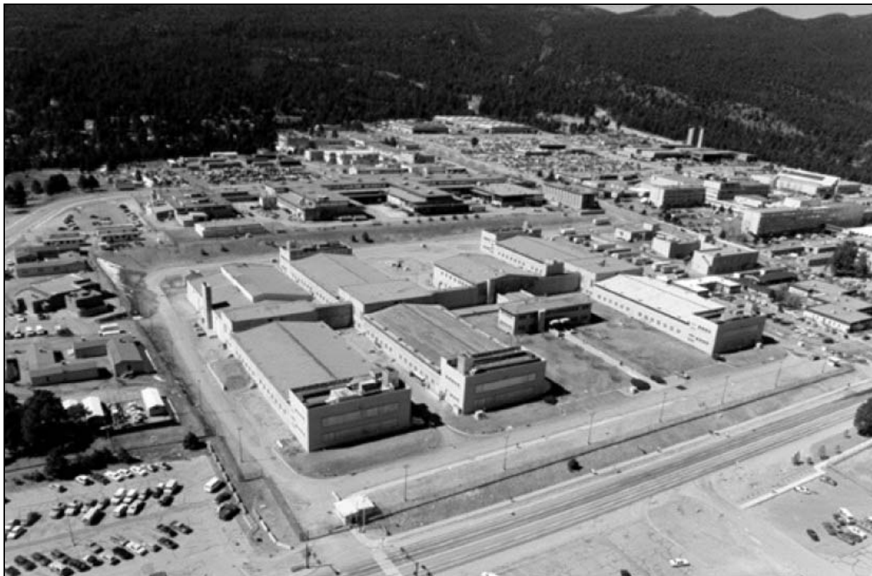
Figure 2–1 Existing Chemistry and Metallurgy Research Building
