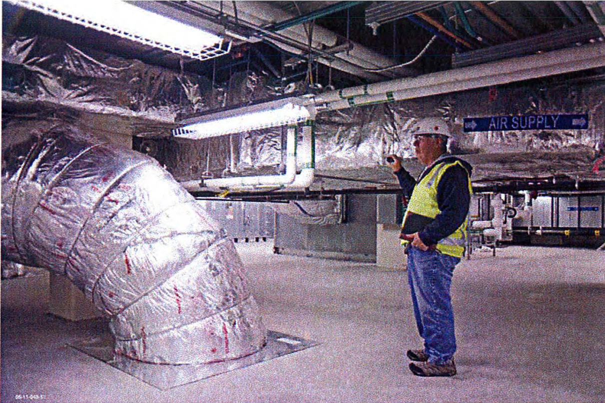
Figure 2–6 Utility System Floorspace in the Radiological Laboratory/Utility/Office Building
