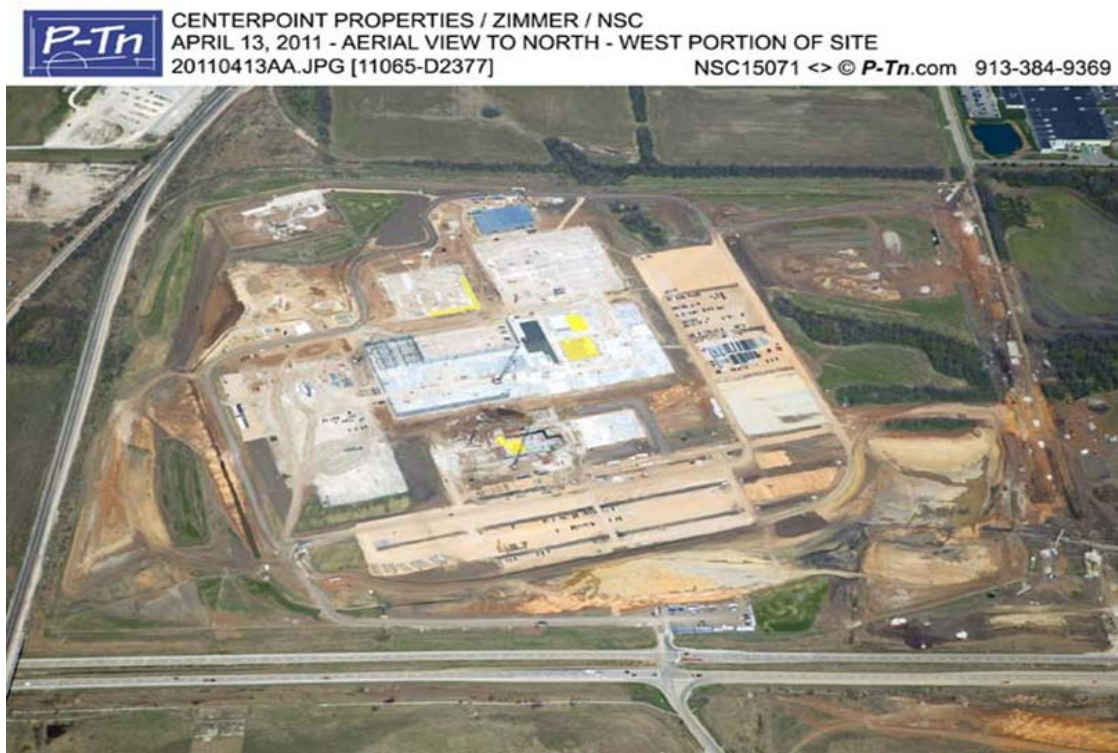
Figure 4: Botts Road Site Construction Progress as of April 13, 2011
