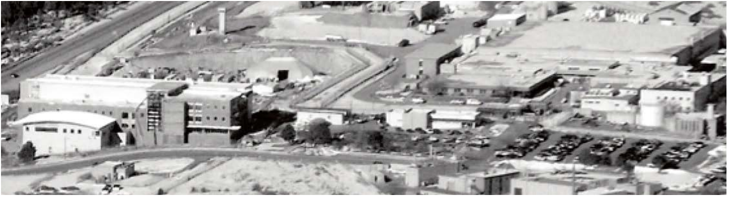
LANL's existing plutonium pit production facility (PF-4) on right, the newly built CMRR Rad Lab on left, with premature excavation for the canceled Nuclear Facility behind it. NNSA is now planning to build underground "modules" between PF-4 and the Rad Lab. Picture credit: Nuclear Watch New Mexico
