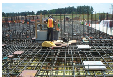
Figure 1-4: WSB Rebar Installed Prior to Basemat Pour
