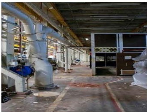
Alpha 5 Facility, post-Recovery Act cleanup effort. (2011)
