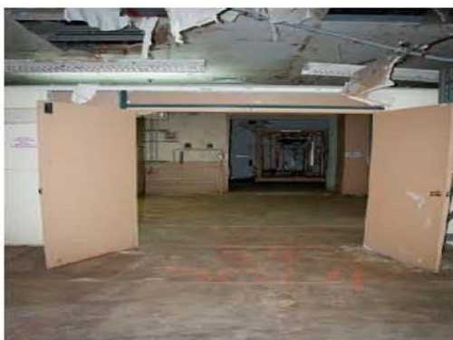
Alpha 5 Facility post-Recovery Act cleanup effort. (2011)
