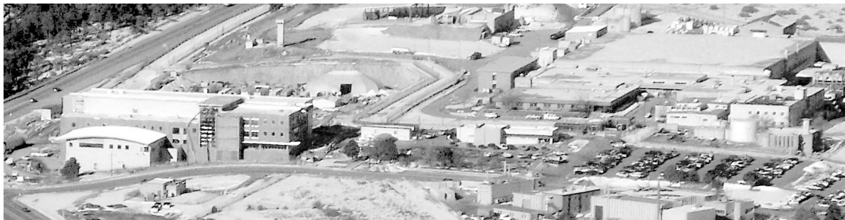
LANL’s Technical Area-55 with the plutonium pit production facility “PF-4” on the right and CMRR “Rad Lab” on the left, with the excavation for the future “Nuclear Facility” behind it. Photo: Scott Kovac, Nuclear Watch New Mexico July 2010
