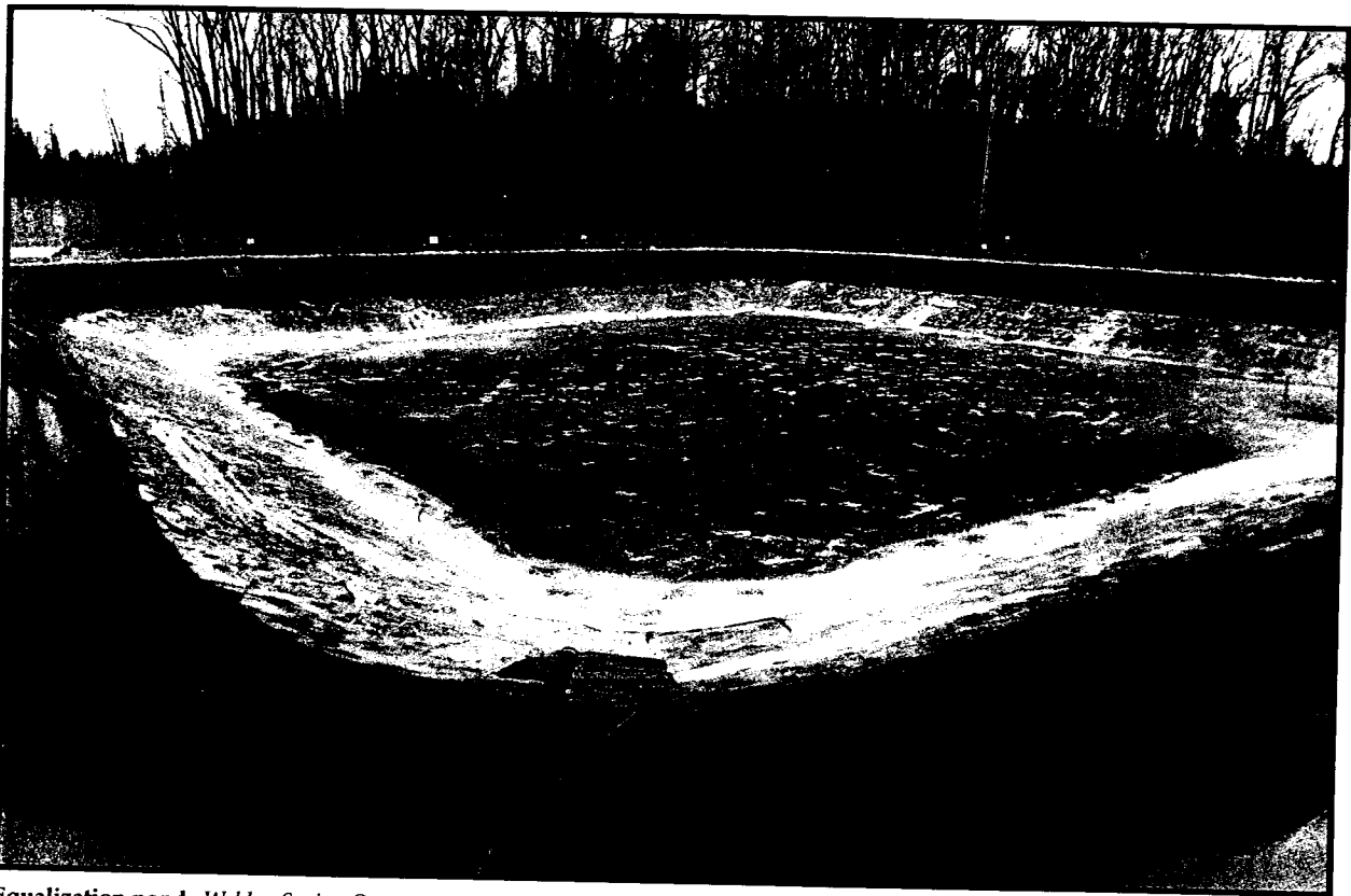
Equalization pond. Weldon Spring Quarry, near the Weldon Spring Site, St. Charles County, Missouri. January 29, 1994.
