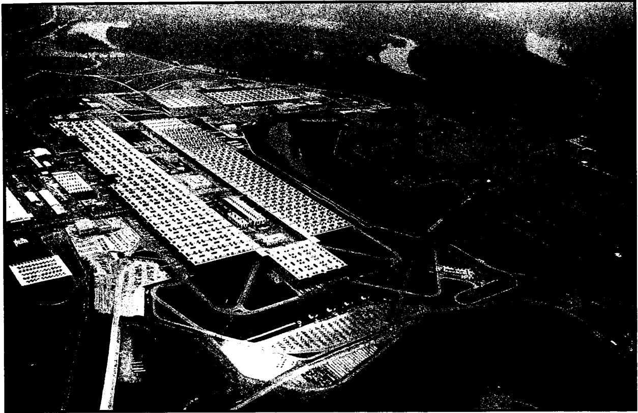
The K-25 Gaseous Diffusion Plant enriched uranium for nuclear weapons and commercial reactor fuel from 1945 until 1987. When first built, the U-shaped K-25 building was one of the largest roofed structures in the world, covering nearly 43 acres. K-25 Gaseous Diffusion Plant, Oak Ridge, Tennessee. June 12, 1982.
