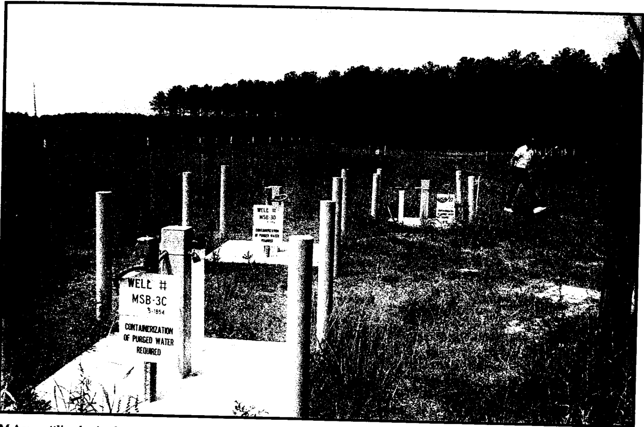
M Area settling basin closure site. Metalworking facilities in M Area fabricated fuel and targets for the Savannah River Site's five production reactors. Wastes discharged to the basin from these processes seeped into the groundwater. The wells in the foreground are part of a groundwater treatment system. M Area Settling Basin, Savannah River Site, South Carolina. June 15, 1993.
