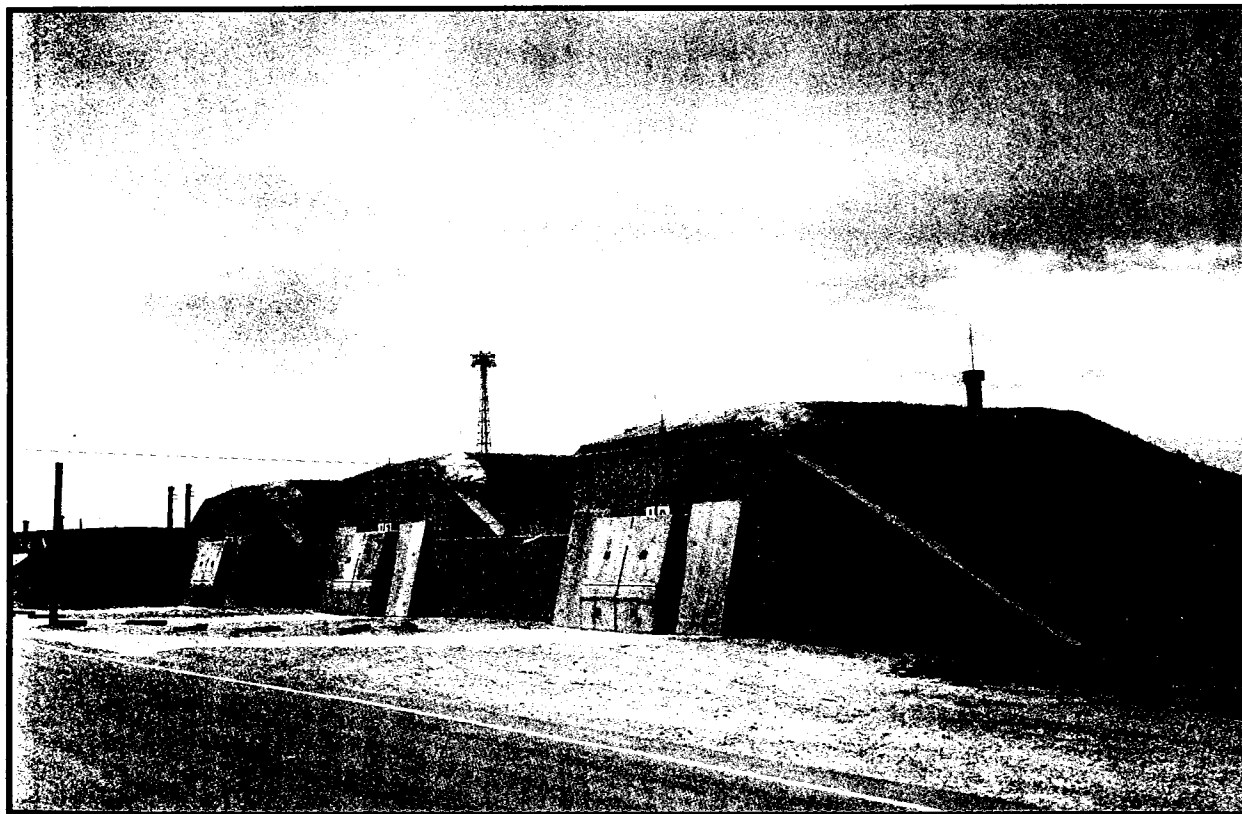
Staging bunkers, or “igloos,” contain nuclear weapons and plutonium pits from dismantled warheads. There are 60 of these earth-mounded bunkers in a high security zone of the Pantex Plant. Sixteen of them store plutonium pits; the remaining 44 house nuclear weapons entering or exiting the plant. Pantex Plant, Amarillo, Texas. May 23, 1986.
