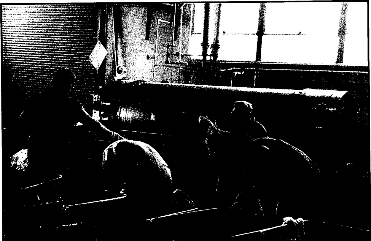
Fernald Laundry. At the Fernald site, over 1,000 pairs of cotton work suits were laundered daily to rid the clothing of uranium dust. Laundry water was treated as low-level radioactive waste because of its uranium content. Feed Materials Production Center, Fernald, Ohio. December 16, 1985.
