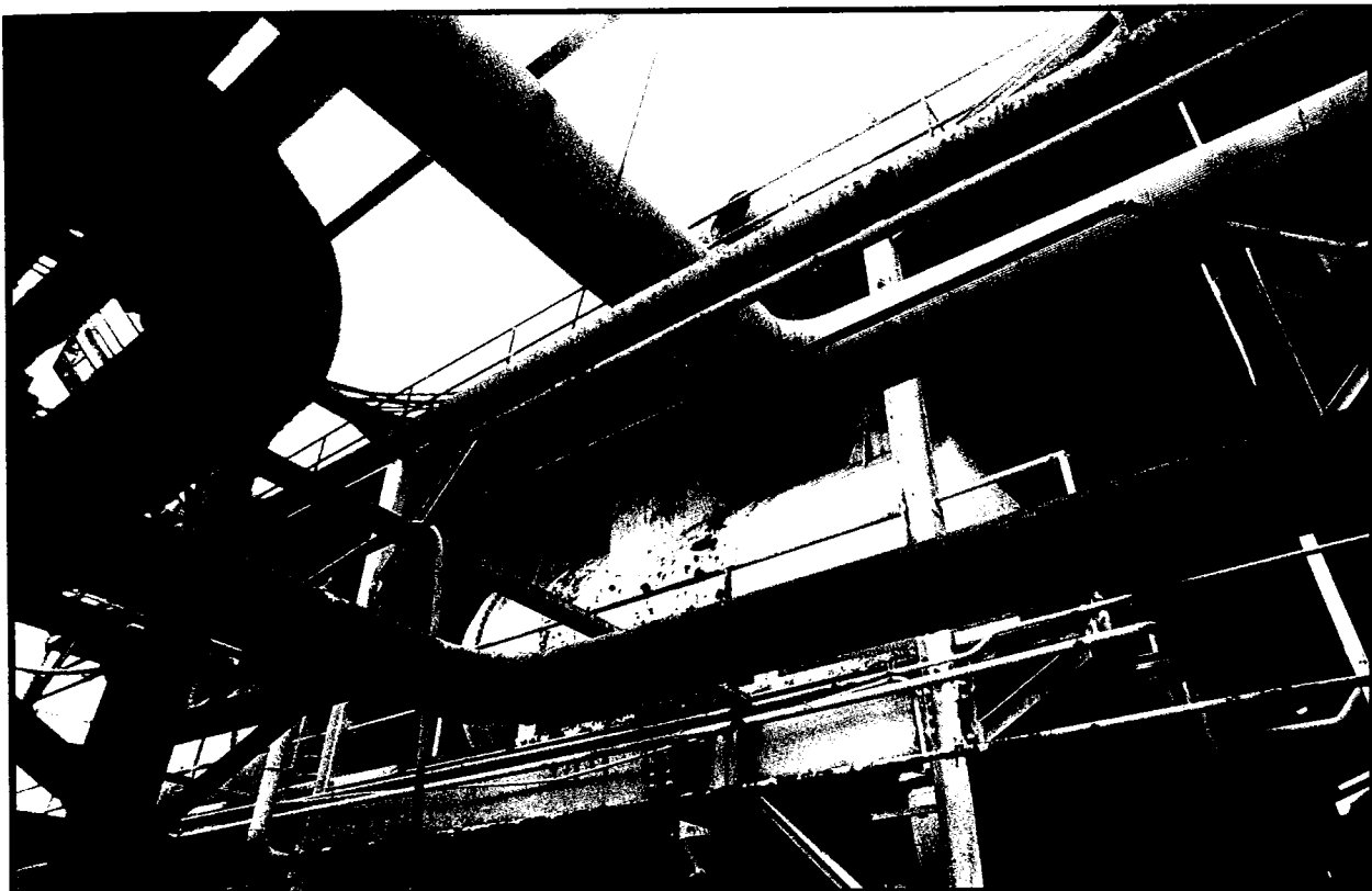
COLEX lithium-enrichment equipment. This plant was shut down in 1963. Alpha 4 Building, Y-12 Plant, Oak Ridge, Tennessee. January 11, 1994.
