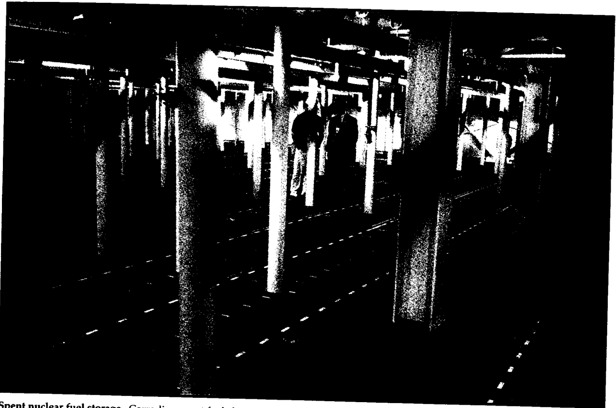
Spent nuclear fuel storage. Corroding spent fuel elements from Hanford's N Reactor are stored in an unlined concrete pool in the 105 K-West area. Steel grates suspended above the surface of the water allow workers to access all areas of the pool. Corrosion of the fuel elements enables radioactive materials to escape into pool water, posing a hazard to workers and the environment. To reduce the danger, the Department is building a new storage facility for this corroding fuel away from the Columbia River. At this new facility, engineers will dry out the spent fuel and store it in special casks to await storage in a geologic repository. 105 K-West Basin, 100 K-Area, Hanford Site, Washington. December 19, 1993.
