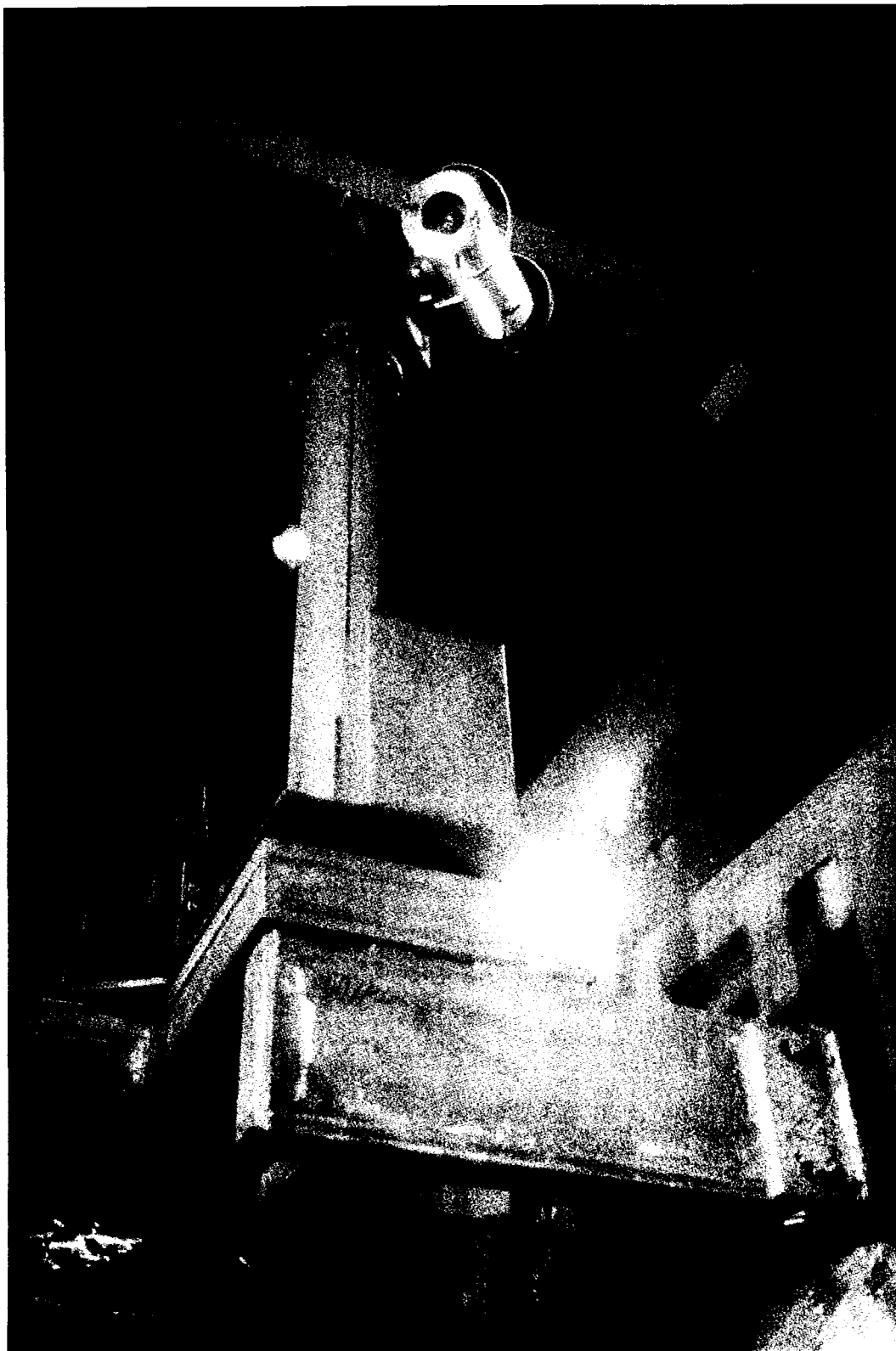
A remote monitoring camera inside the Defense Waste Processing Facility allows workers to monitor operations in the world's largest high-level nuclear waste processing facility. This facility fills canisters with high-level nuclear waste solidified in glass. The waste was generated by reprocessing operations, which extracted plutonium for use in nuclear weapons. The waste-filled canisters are stored awaiting the availability of a geologic repository for permanent disposal. Savannah River Site, South Carolina. June 15, 1993.
