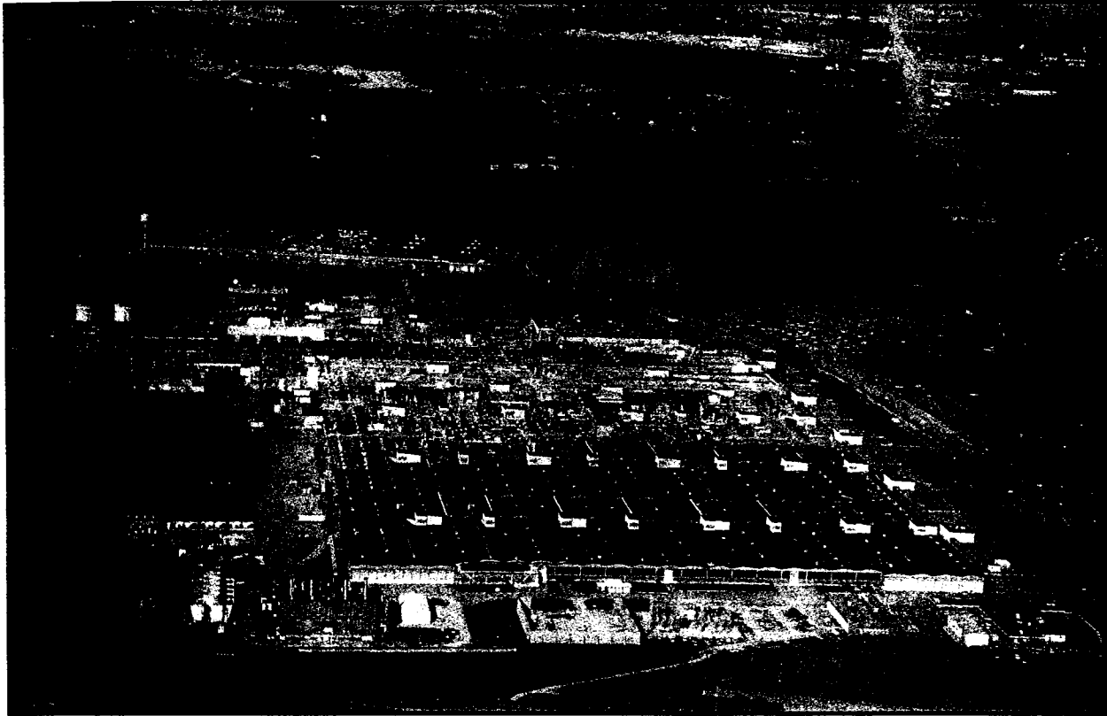
The Kansas City Plant manufactured nonnuclear components for nuclear weapons. Since 1949, its products included arming, fuzing, and firing systems, radars, power supplies, rubber, plastic and foam parts, and outer casings. This plant is now DOE's only facility for manufacturing nonnuclear components for nuclear weapons. Kansas City Plant, Bannister Federal Complex, Kansas City, Missouri. July 17, 1982.
