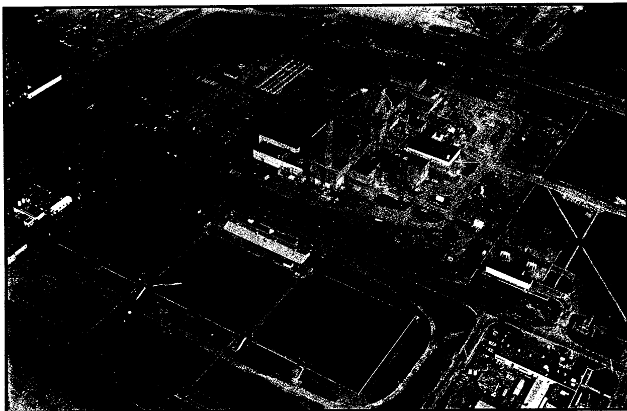
L-Reactor, Savannah River Site. Mark 31 target cores from Fernald were loaded into this reactor and bombarded with neutrons, which transformed some of the depleted uranium metal into plutonium. In front of the reactor are three reservoirs of cooling water. The Savannah River Site had a total of five plutonium production reactors. L Area, Savannah River Site, South Carolina. August 6, 1983.
