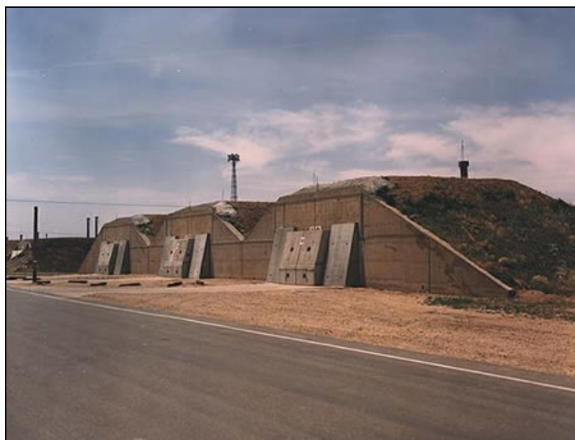
Figure 3.7-3 — Typical Storage Igloos at Pantex
