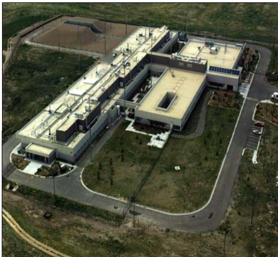
Figure A.6.1-6 — Explosives Component Facility (ECF); SNL/NM Bldg 905
