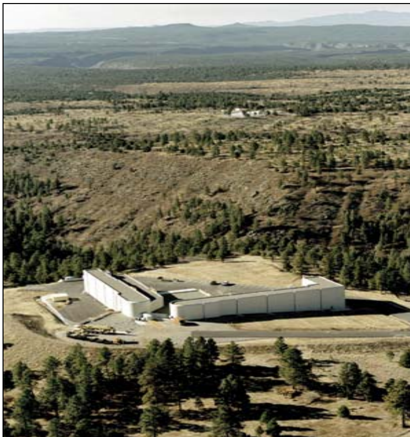
Figure A.9-4 — The DARHT at LANL
