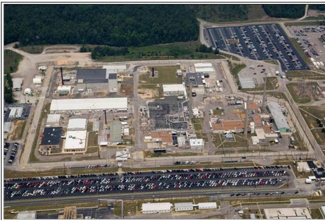
Figure A.7.1-3 — Aerial Photo of SRS Tritium Facilities
