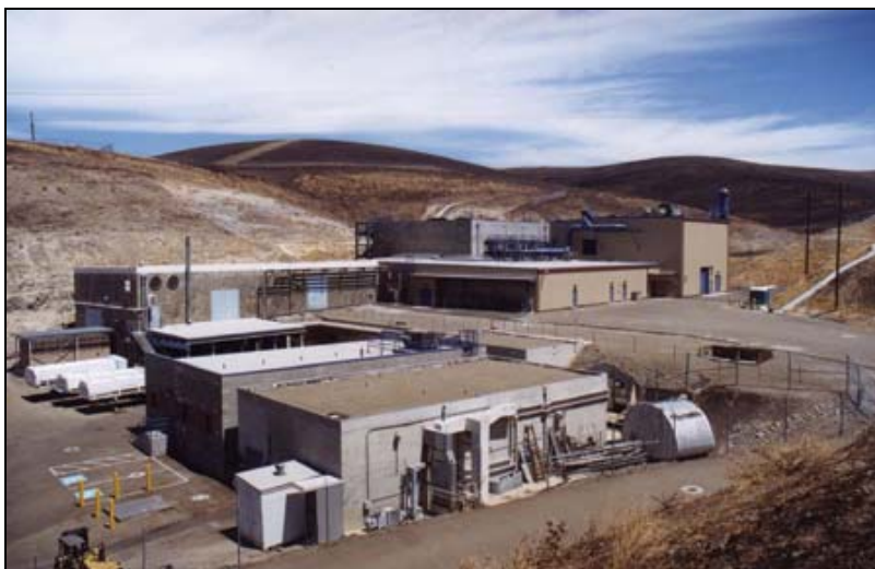
Figure 3.11-2 — The Contained Firing Facility at the LLNL Site 300 Building 801 Complex
