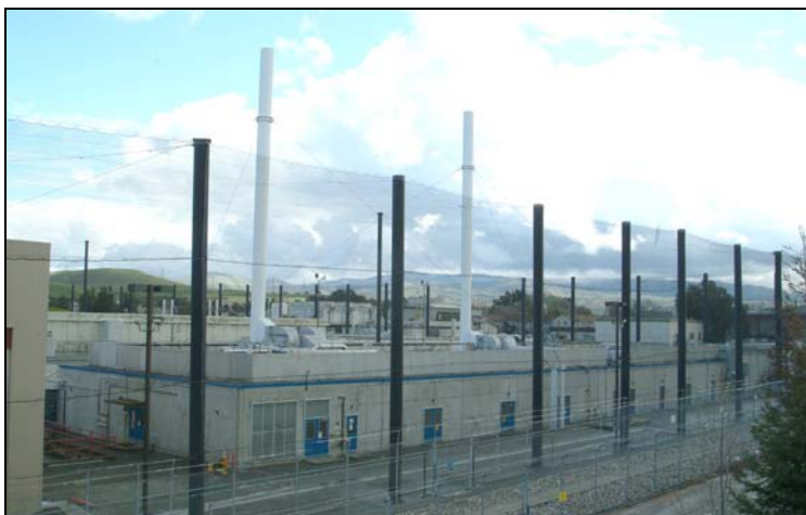
Figure 3.9-1 — LLNL Tritium Facility
