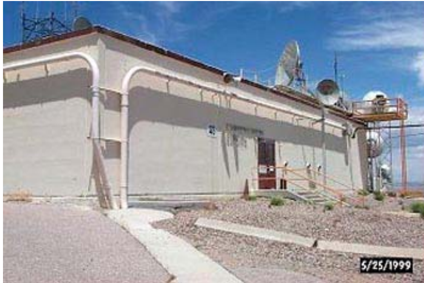
Figure A.8-5 — CP-40 includes administrative areas and a high bay that would be useful for personnel and assembling test hardware
