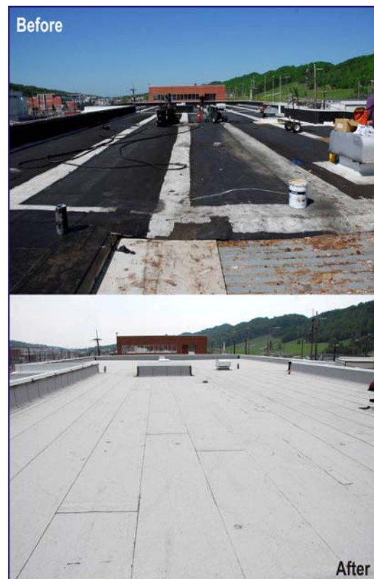
Figure A-11-2. Roof repairs on Building 9113 at Y-12. FIRP replaced 21,300 square feet of roofing on time and within budget.
