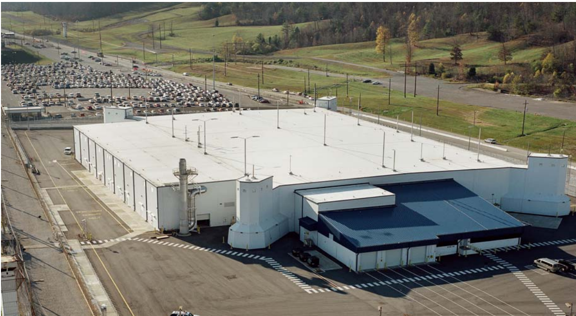
Figure A-8-4. Newly completed Highly Enriched Uranium Materials Facility (HEUMF) at Y-12.
