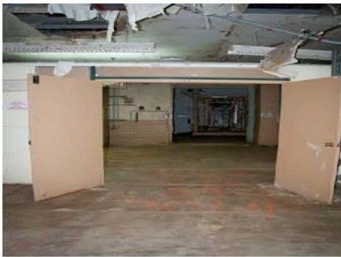
Alpha 5 Facility post-Recovery Act cleanup effort. (2011)
