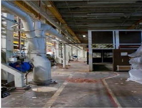
Alpha 5 Facility, post-Recovery Act cleanup effort. (2011)
