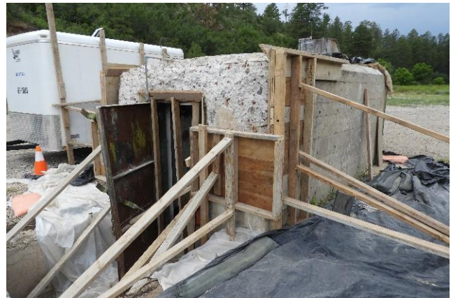
Figure 3-3. Bunker 18-5 during concrete restoration in July 2019
