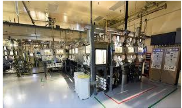
PF-4, LANL's main plutonium facility
