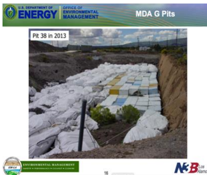
Waste disposed at Area G nears the surface of the 65-foot-deep Pit 38.
